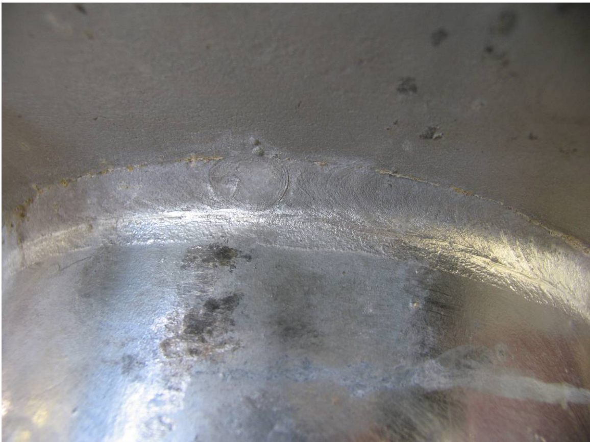
Figure 6.23 Base Plate to Pole Wall Fillet Weld on Run-Out Specimen
