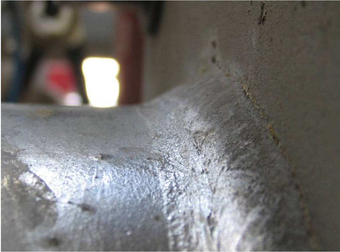
Figure 6.24 Detailed View of Base Plate to Pole Wall Fillet Weld
